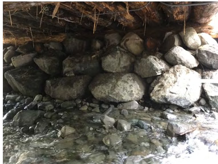
Right Bank Abutment when facing downstream
