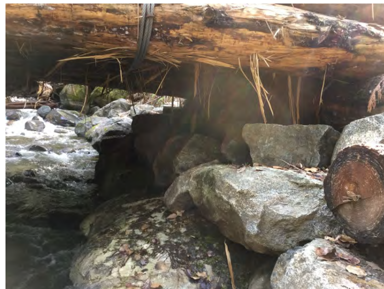
Left Bank Abutment when facing downstream
